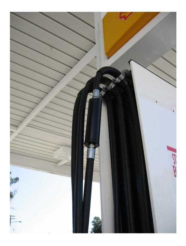
Typical FitSafe or Wix Filter Installation
