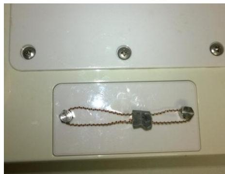
(a) Lead and Wire Type Sealing Arrangement
