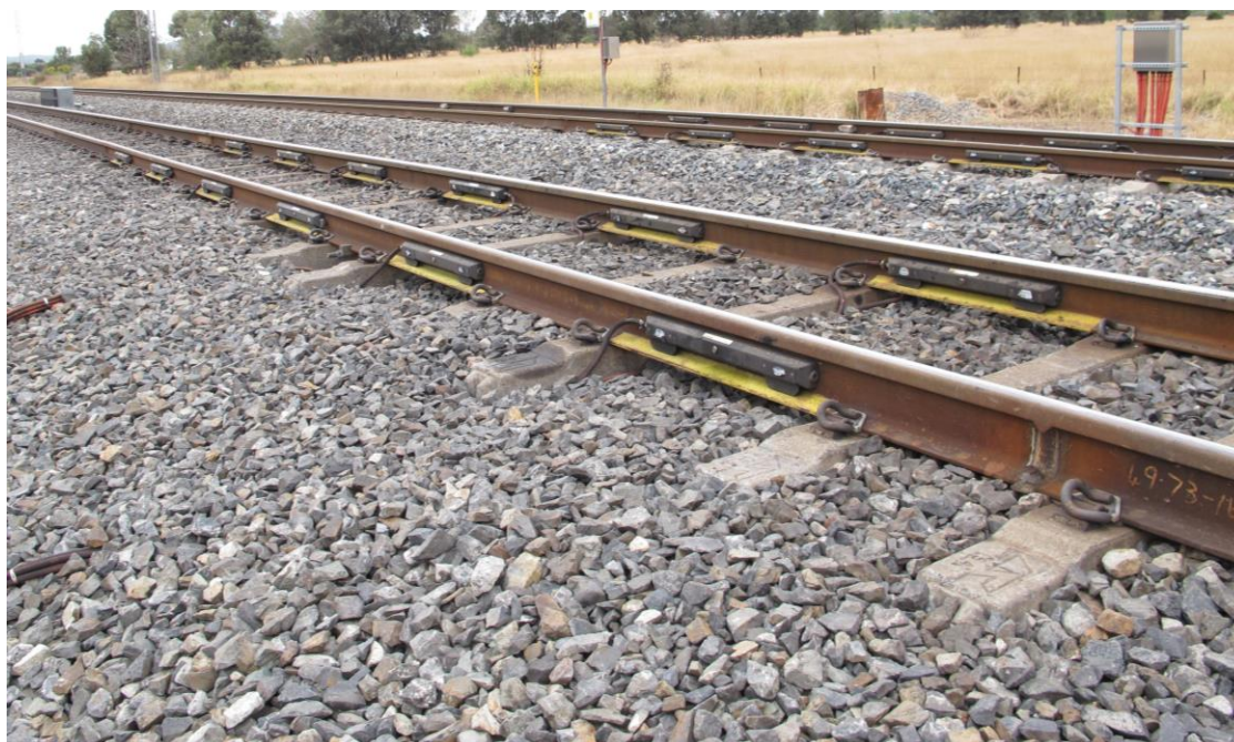
Railweight Model STREAMLINE Model STRMLNAU16 Transducer Installation
