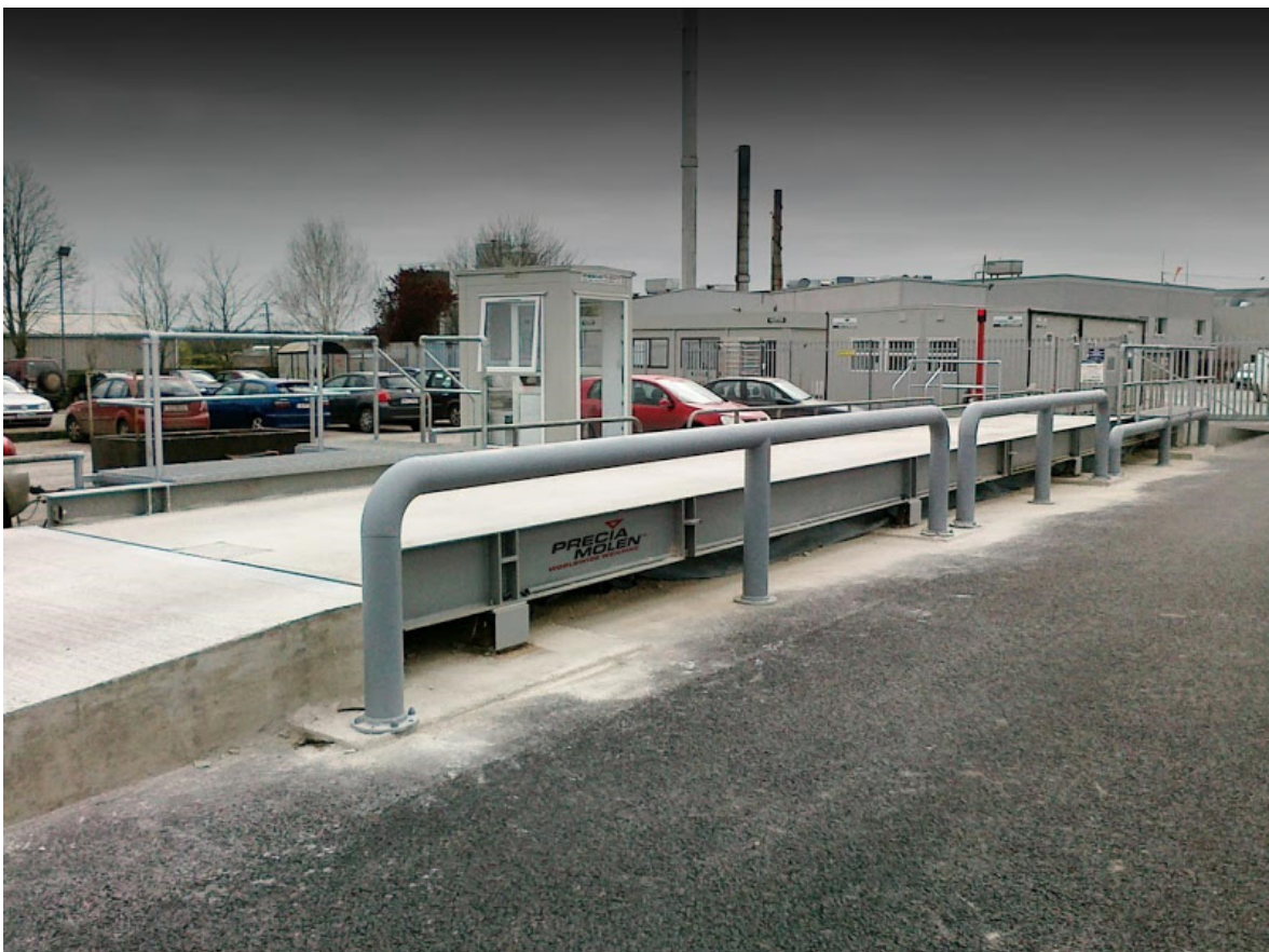
Typical Model SPWB Weighing Instrument - Steel Frame and Concrete Deck
