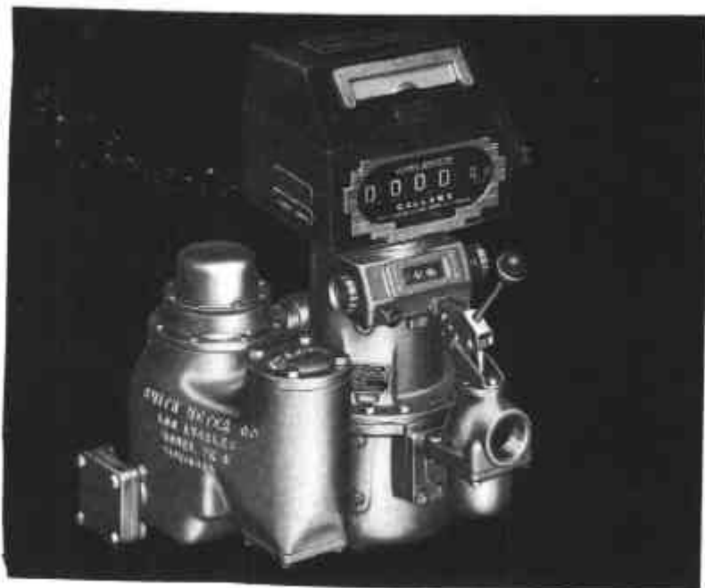
FIGURE 1. Wayne-Smith Flowmeter Model T6
