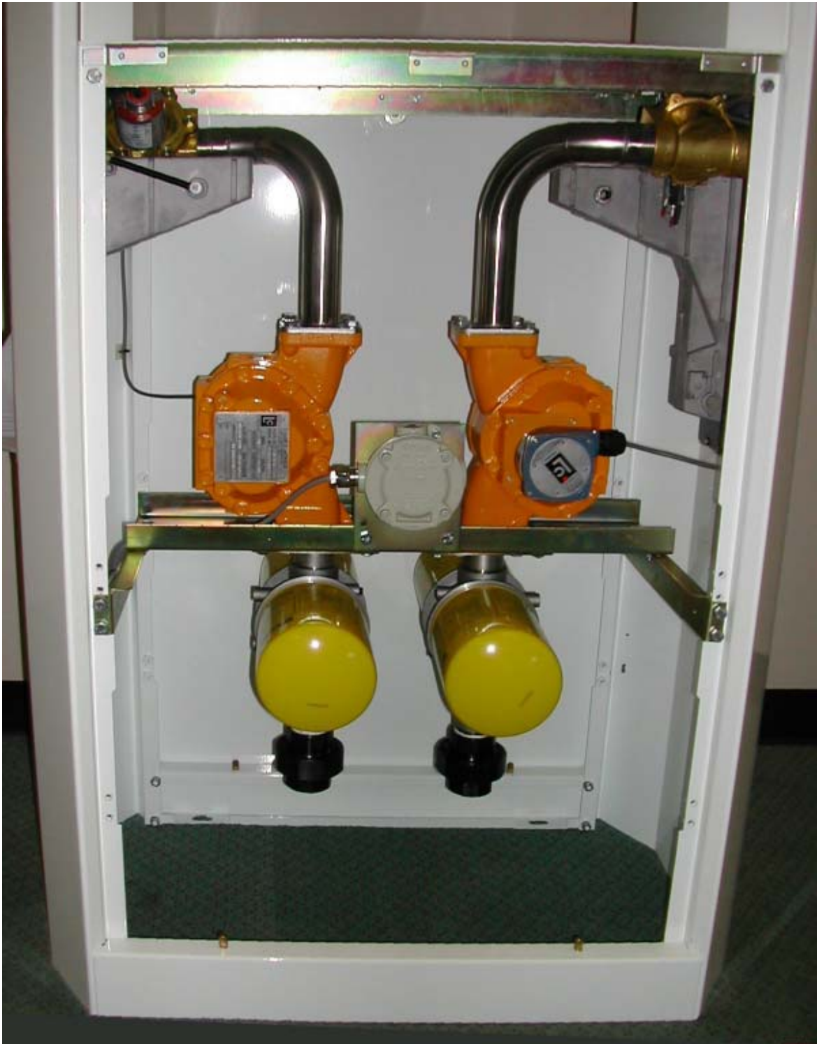
Typical Two Inlet/Two Outlet Fuel Dispenser and With Fuel Supplied From STP Hydraulic System
