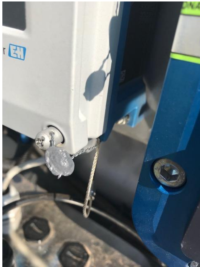
Sealing of Promass 300 Transmitter
