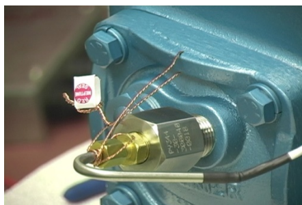
Sealing of the Temperature Probe Installed on the Red Seal Gas Purger
