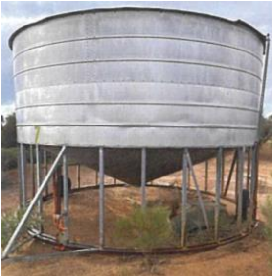
Picture 3. This picture shows an older silo made from ALLGAL® square tube with the zinc coating completely gone on the base ring and substantial corrosion on the legs compared to pipe frame silos.
