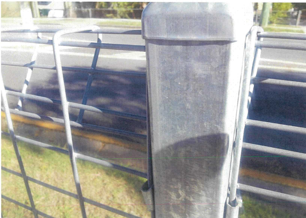
Photo 4 – Close up picture of pre-galvanised SHS fence showing weld repair strip on left hand side of product
