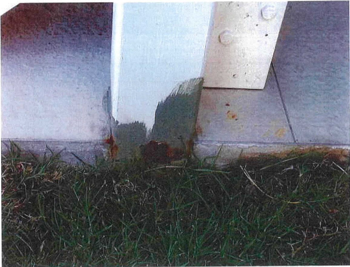
Corrosion in a steel post
