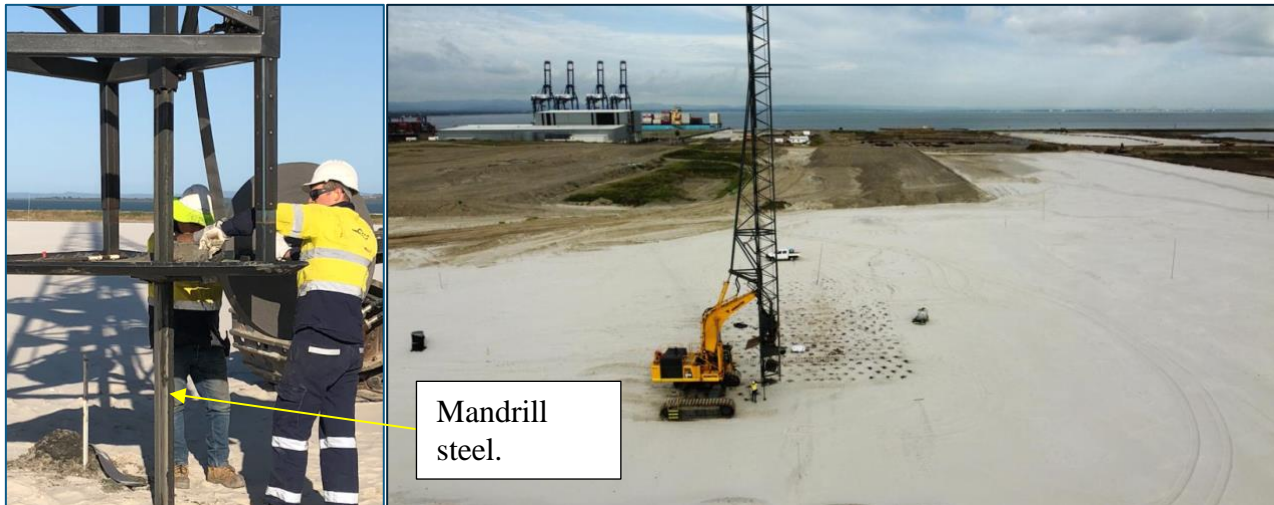
MGN Civil Wicking Rig, highlighting the required mandrill steel.
