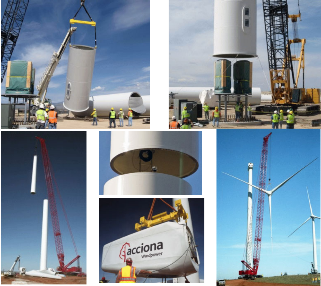
Figure I-7 Wind towers: Turbine installation
