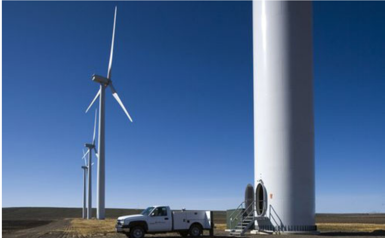
Figure I-3 Wind towers: Installed wind turbines
