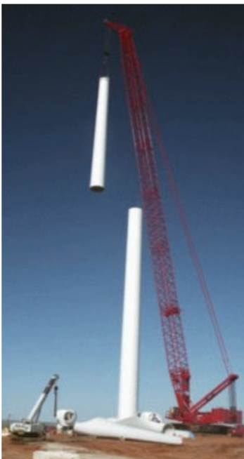
Raising and positioning the next tower section over those already in place.
