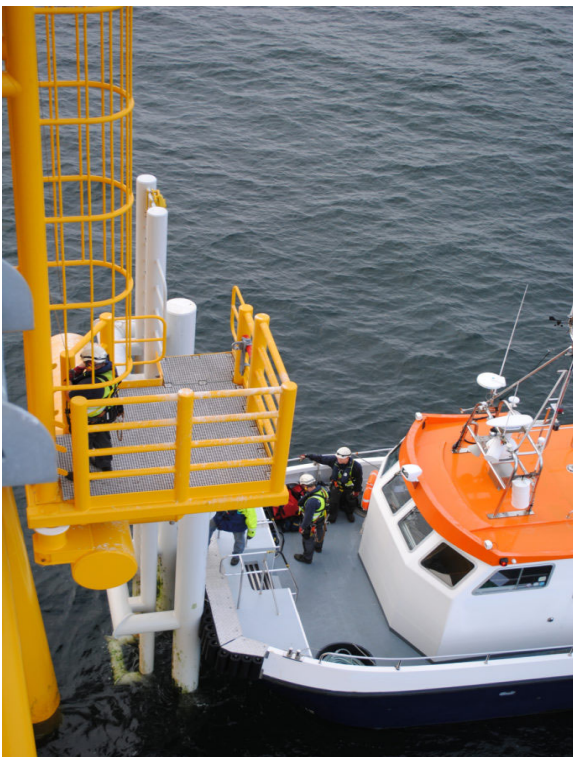
Transition piece with mooring fixture and ladders.
