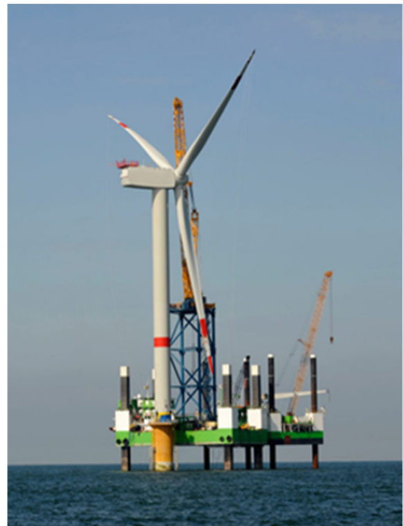
Installing the rotor assembly onto the nacelle.
