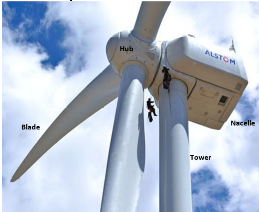
Figure I-1 Wind towers: Utility-scale wind turbine
