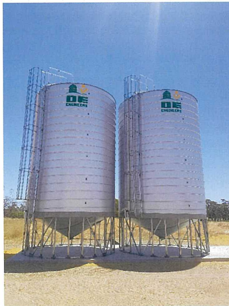
Picture A: Silos set up on concrete pads
