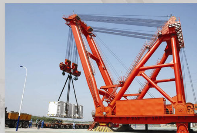
800T码头吊装 800T wharf hoisting
