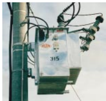
315 kVA 22 kV pole-mounted transformer with galvanised tank
