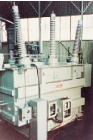
100 MVA 220 kV power transformer
