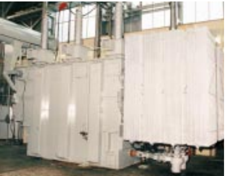
60 MVA 132 kV power transformer
