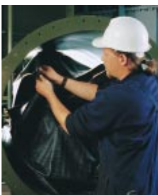
Fitting conservator oil preservation system
