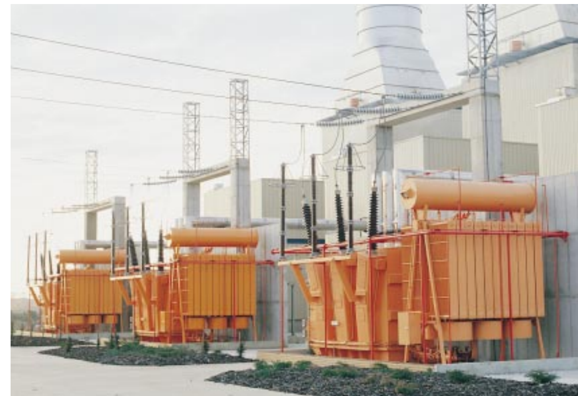
220 kV generator transformers
