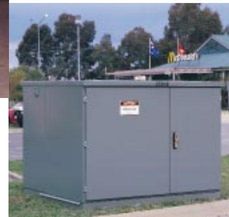
Pad-mounted substation
