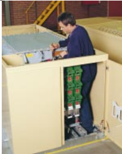
Compact substation fit-out
