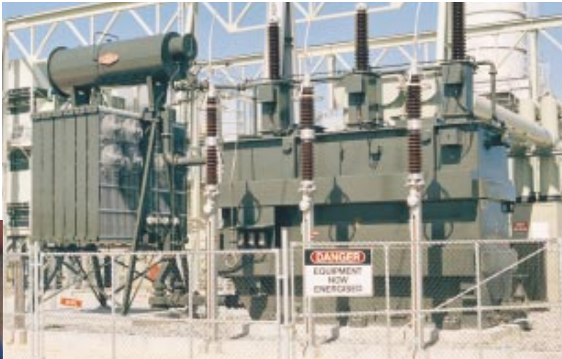
140 MVA 132 kV generator transformer
