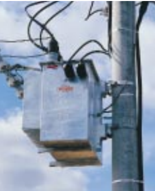
315 kVA 22 kV pole-mounted transformer
