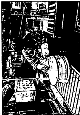
Mechanical fettling for cosmetic appearance.
