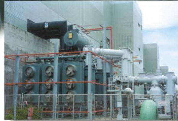
345kv 250MVA Power Transformer for Combustion Power Plant
