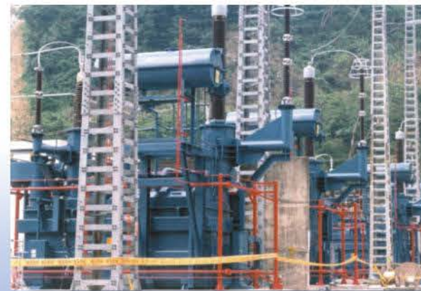
345kv 500MVA Power Transformer for EHV Substation
