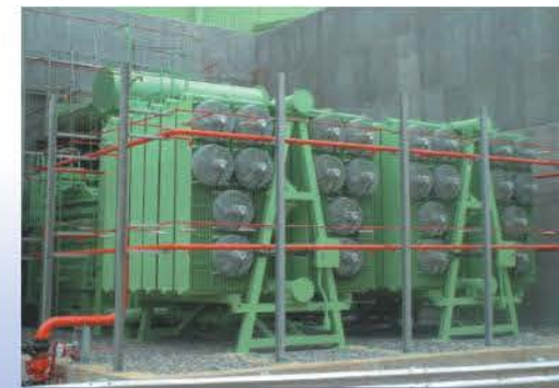
161kv 290MVA GSU (Generator Step-up Power Transformer) for IPP
