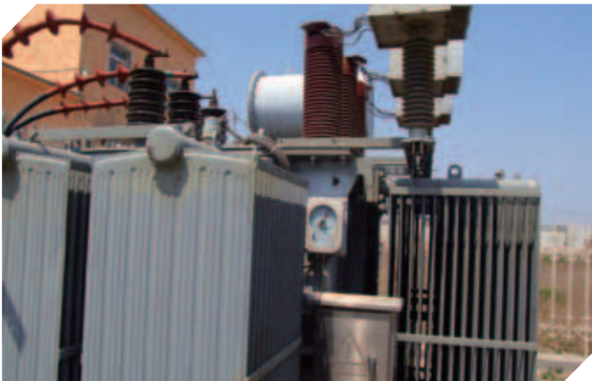
Yuedong Oilfield: Power compensation device
