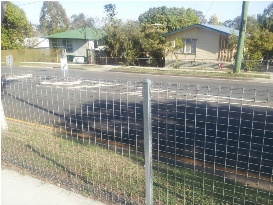
Photo 3 – Picture of fence with pre-galvanised SHS as posts
