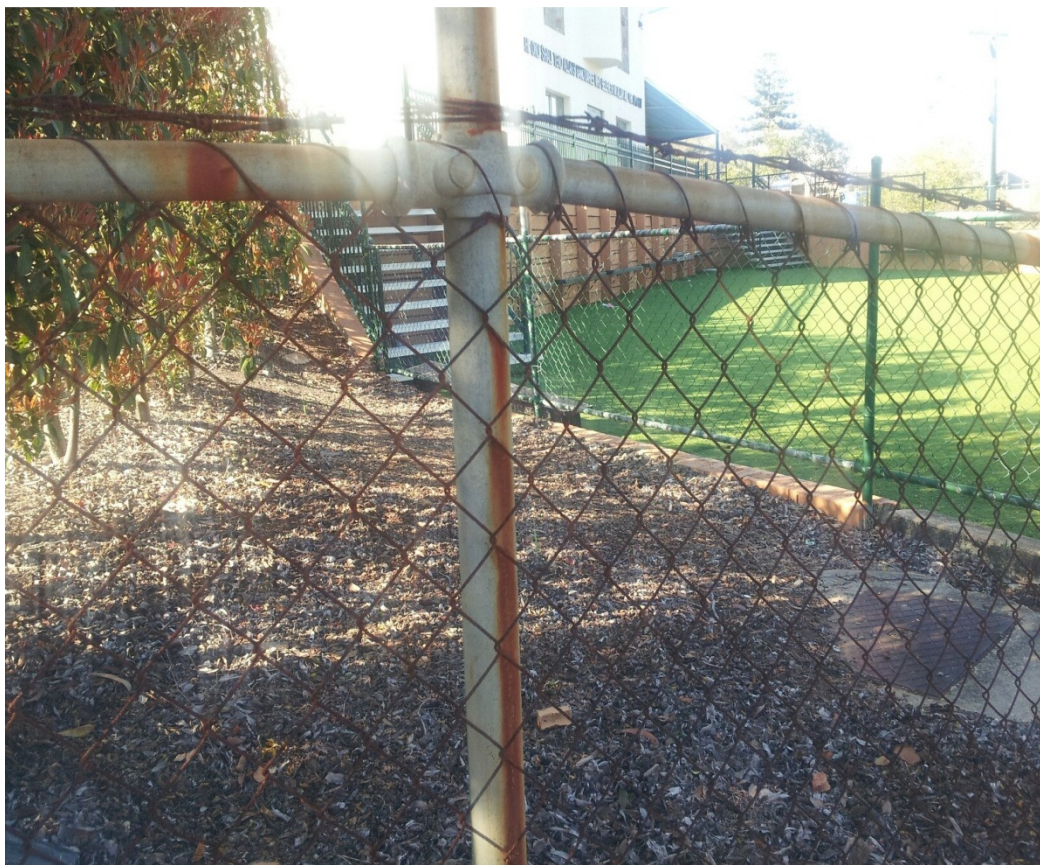
Photo 2 – Close up picture of fence with HDG air blown pipe as posts
