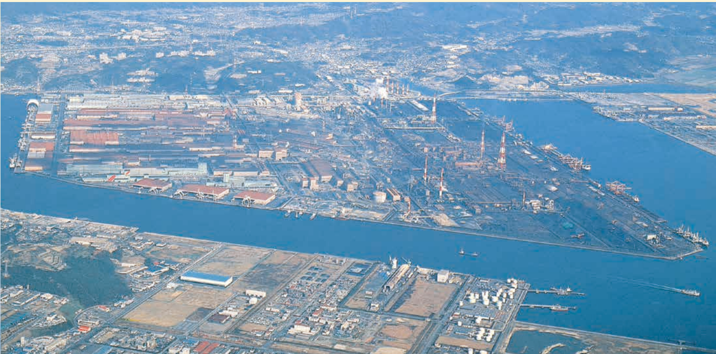
West Japan Works (Fukuyama)
