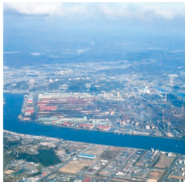
▲ West Japan works (Fukuyama)
