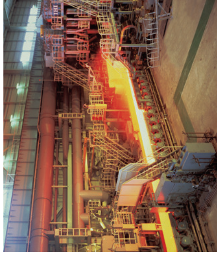
No. 3 hot strip mill line of East Japan Works (Chiba District)
