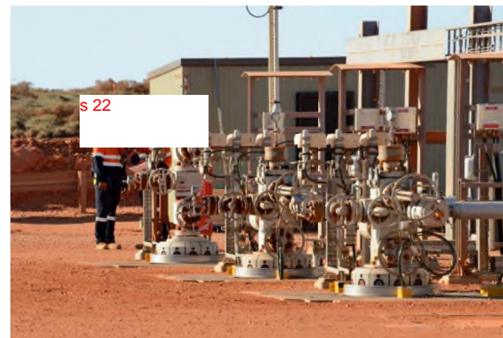
Figure 4: Three of the wells (surface trees) at injection drill centre A.
