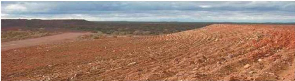
**Gambar 5.26 - Lereng cekung timbunan limbah di Murrin Murrin**
